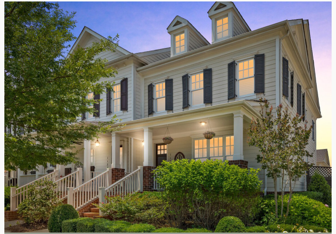
1121 WESTHAVEN BOULEVARD | FRANKLIN
