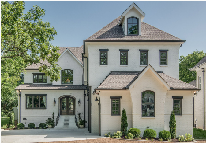
3823 TRIMBLE ROAD | NASHVILLE
